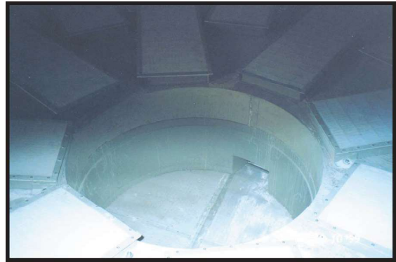
Aerated bin bottom silo discharge.
