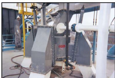
Aerated distribution box with four discharges.
