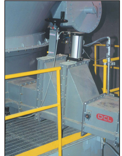
Vertical manual and pneumatic slide gate valve.
