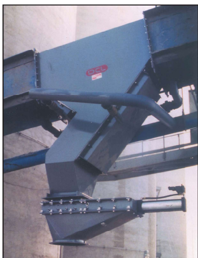
Aerated lump trap with slide gate valve.
