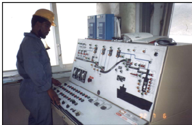
Fig. 3c. New 'DCL' console controls all equipment from storage reclaim to ship loader.
